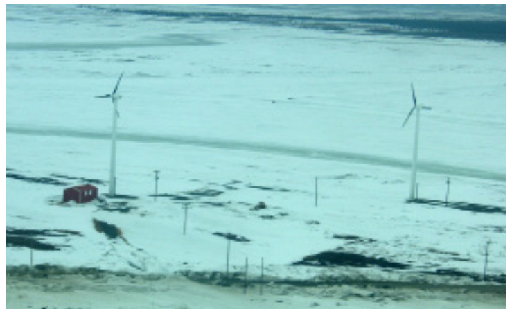
Northern Power 100B turbines, photo courtesy of Solsticeak.com
